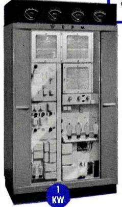
Not only a transmitter in itself, this unit serves as the basic driver for all higher powered transmitters.
