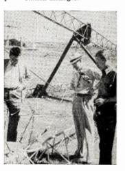
AN 80-MILE wind sheared off at its base the smaller of two radio towers at KFYR Bismarck, N. D., Aug. 1. Ivar Nelson, station's chief engineer, said the 346-foot tripod was a total loss, although the 704-foot main tower was undamaged. Others are Burt M. Adams, NBC station relations, New York, and F. E. Fitzsimonds, KFYR manager.
